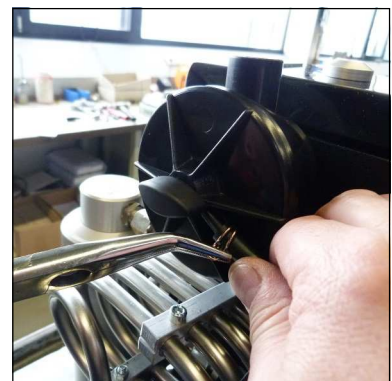
Fig. 7 - Fix spring wire clamp
